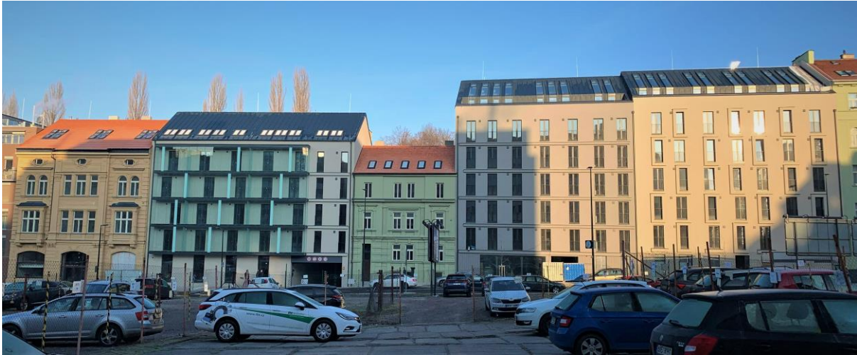
View of the building from Koněvova Street (© PORR)
