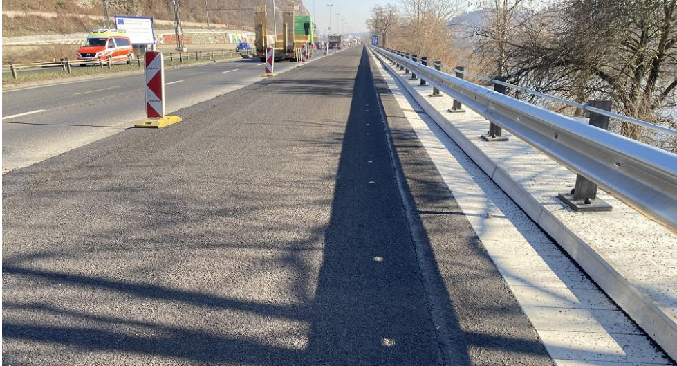
Caption: Completed bus lane on Strakonická street (© PORR)
