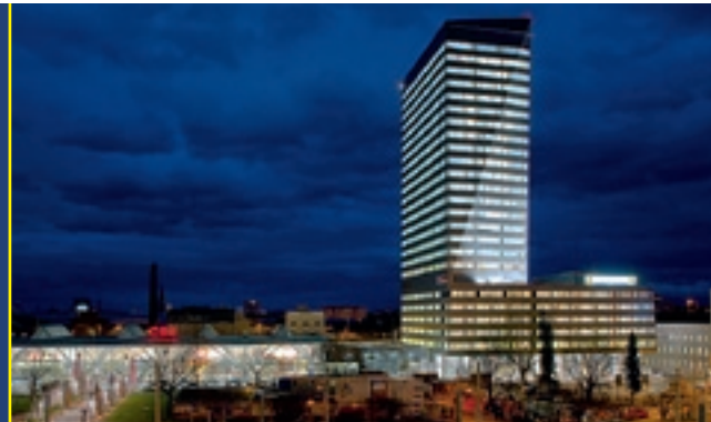
At Linz main railway station, the office tower Terminal Tower was developed and built along with underground parking. The low building consists of an underground level with seven further storeys, on top of which the 18 high-rise floors can be found.
