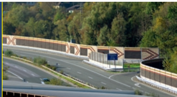
The approx. 3.8 km-long noise barrier , near Deutschfeistritz on the S 35 Brucker motorway, not only meets medical recommendations, but also technical and aesthetic demands.
